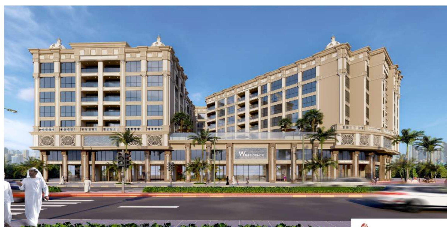
Project: G+P+6F Residential Building Location: Muwaileh, Sharjah, UAE Client: W Residency Consultant: Al Nahda Engineering Consultant Status: Completed
